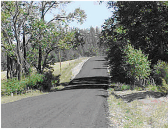
Montana pugmilled and grader placed RAP.
